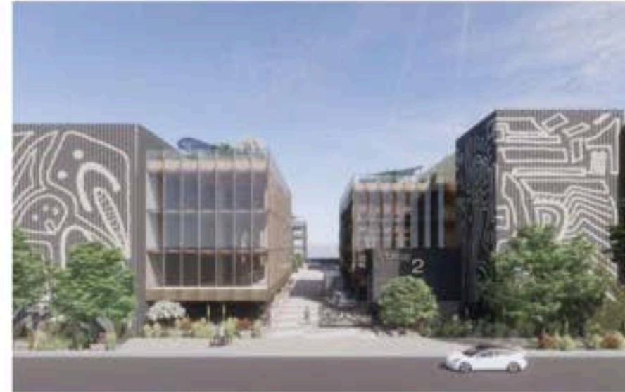
View of Base Camp Alley and Support facilities
