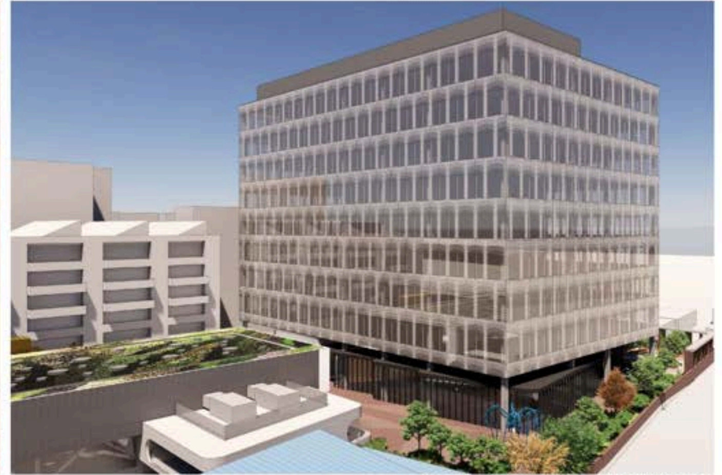
Overview of the nine story building and production studio buildings
