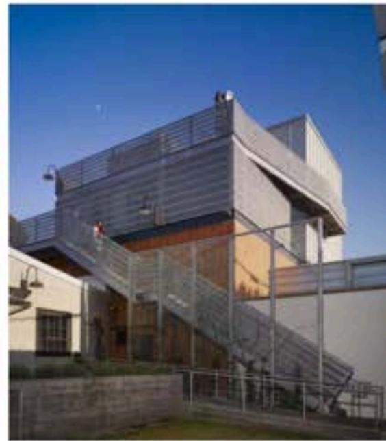
Access to the Roof Deck and Tower
