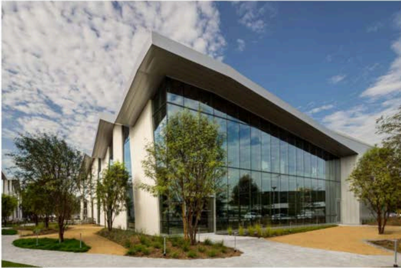
View of building entry
